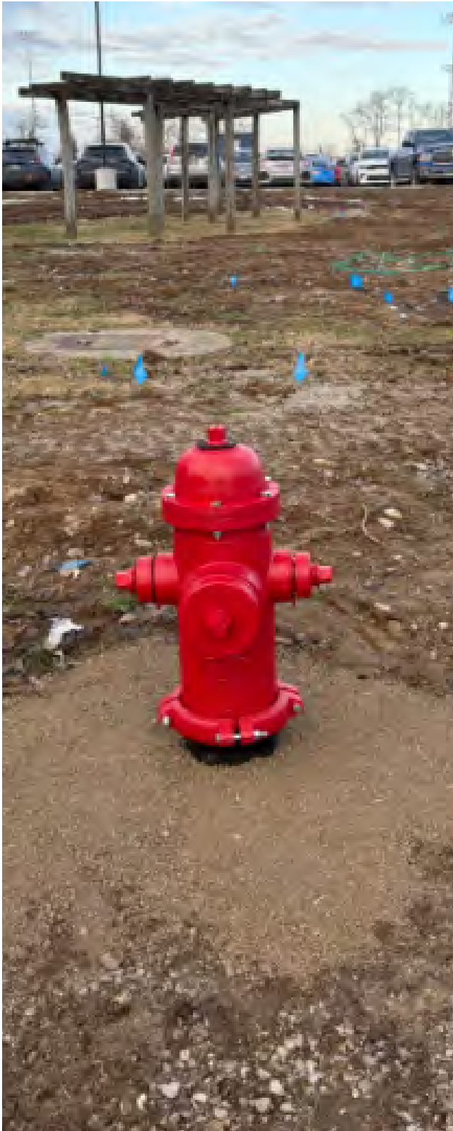
Two newly refurbished fire hydrants.
